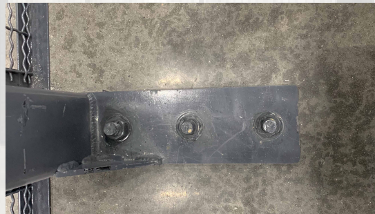
Welded on base plates for lagging to floor
